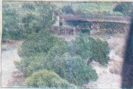
This is how the bridge in the Lusushwana river in Matsapha looked like.
