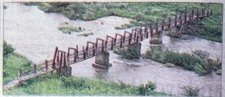
Tebetebe was not damaged at Mpuluzi.
